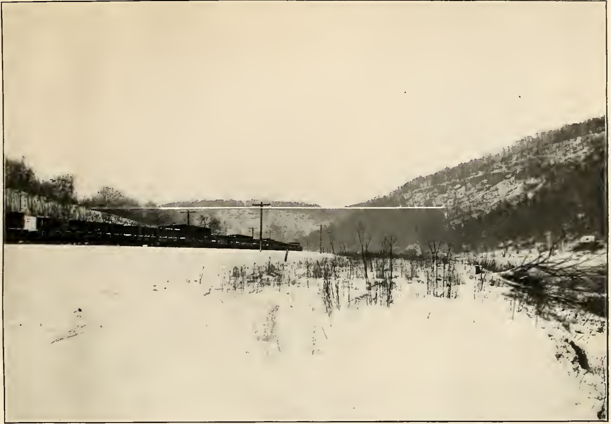
ALLEGHENY RIVER, PA., FEBRUARY, 1911. View up stream, showing crest of proposed Dam No. 1.
